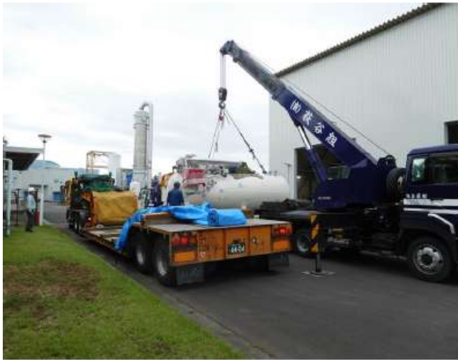
Loading of Cold box
