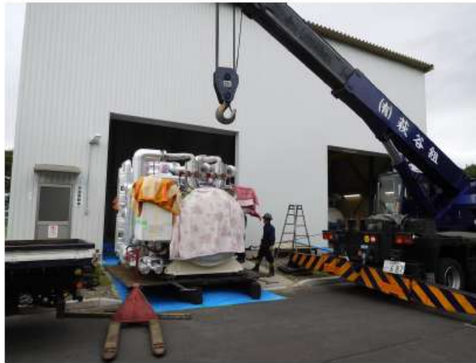
Installing of Cold box
