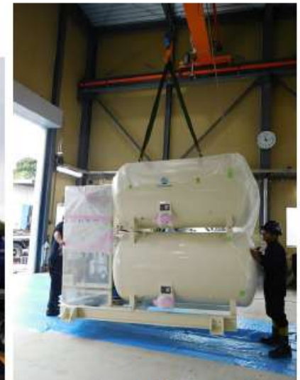
Installing of Gas charge unit
